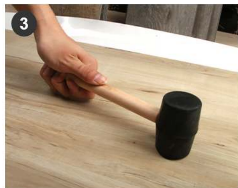
Use a soft-faced hammer to lock planks on the short side
