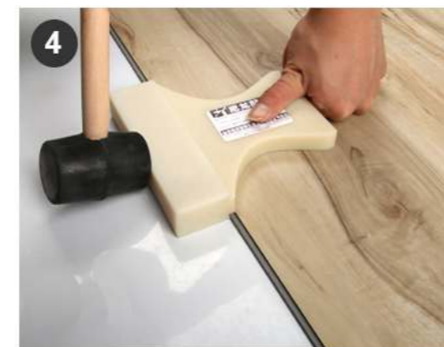
Use a soft-faced hammer to properly lock the planks
